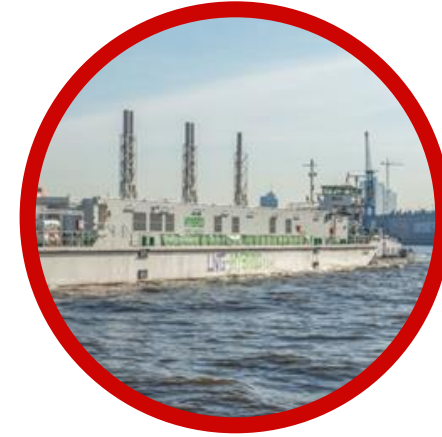
Floating liquid gas power plant LNG Hybrid Barge "Hummel"
