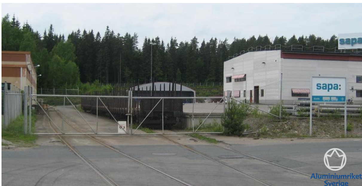
Figure 23 The Aluminum terminal in Vetlanda need to bed extended in order to handle increased freight volumes (Photo: Fredrik Bärthel, Vectura).
